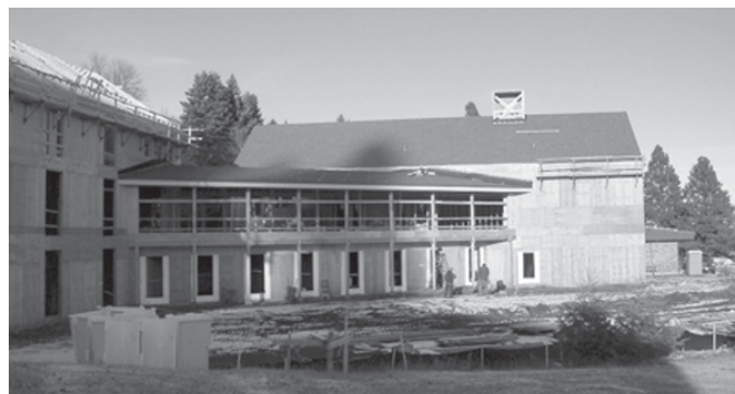
Some roofing is complete and window installation is beginning.
